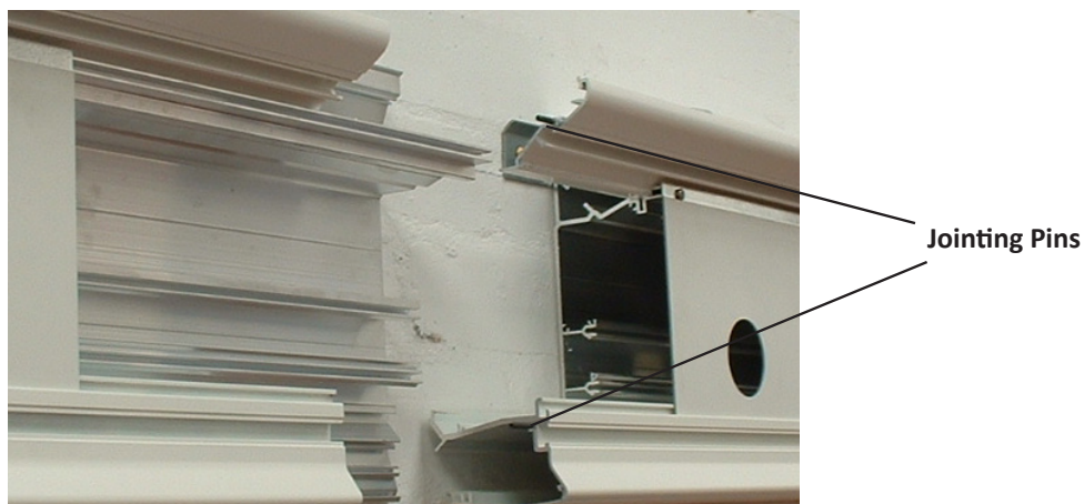
Figure 3 – Preparation for Trunking Joining
