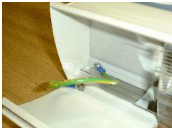
Installation of 16mm 2 earth cable
