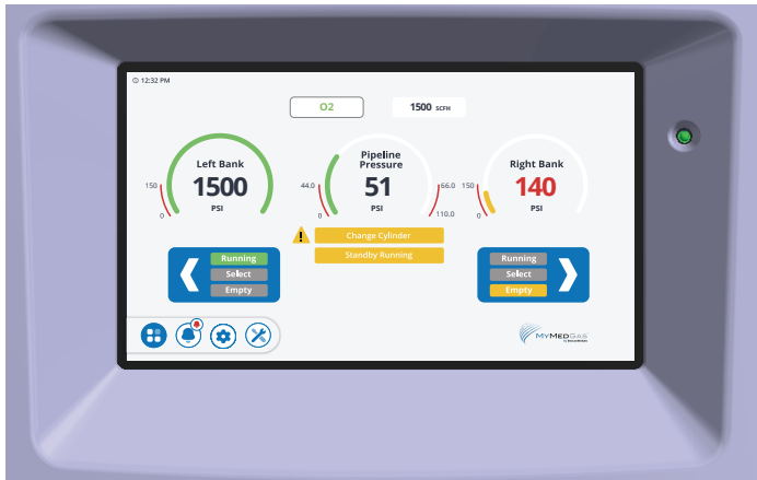
Figure 20 - Right Bank Low, Left Bank Running.
