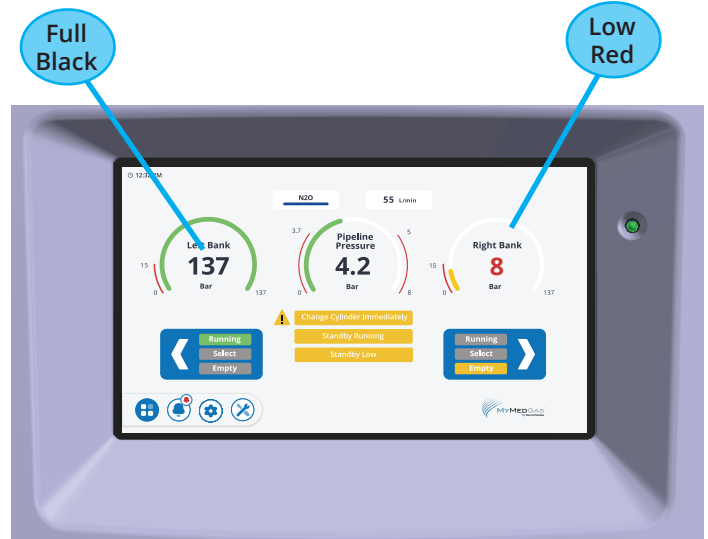
Figure 28 - Left Bank Running, Right Bank Empty.
