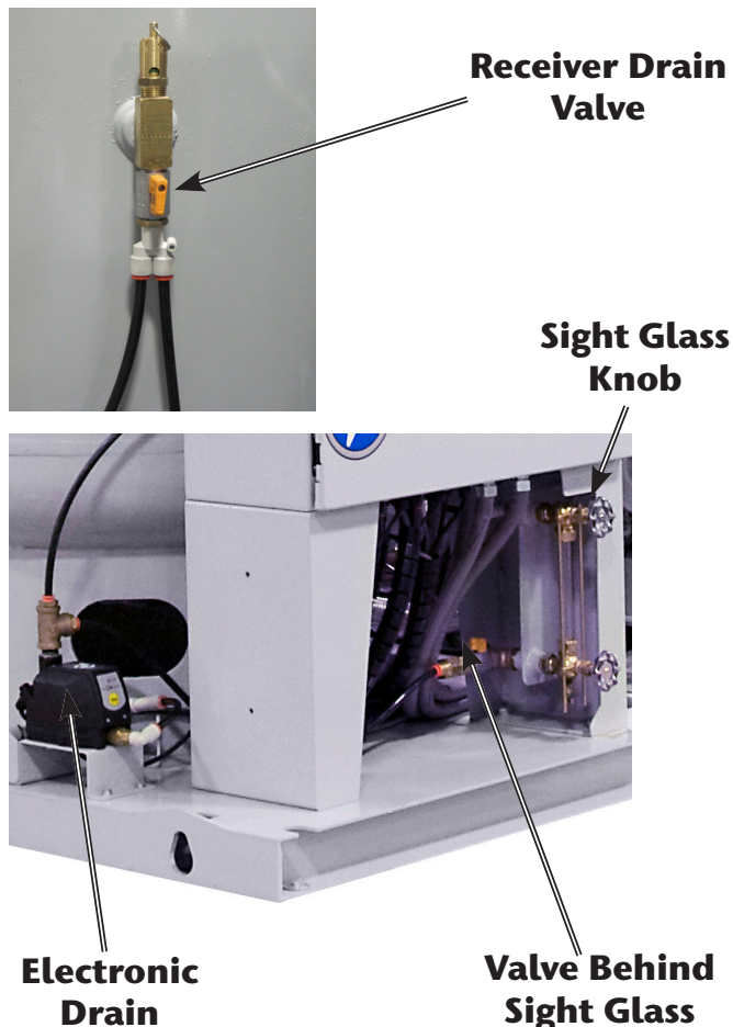
Figure 6.5.1.1 Electronic Drain Isolation Valves
