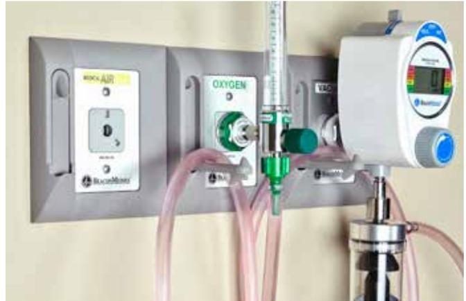
Hook plates take the loads off the outlets, maximizing their longevity and ensuring costly gas leaks are minimized. Simply speaking, the hook plates save you money.
