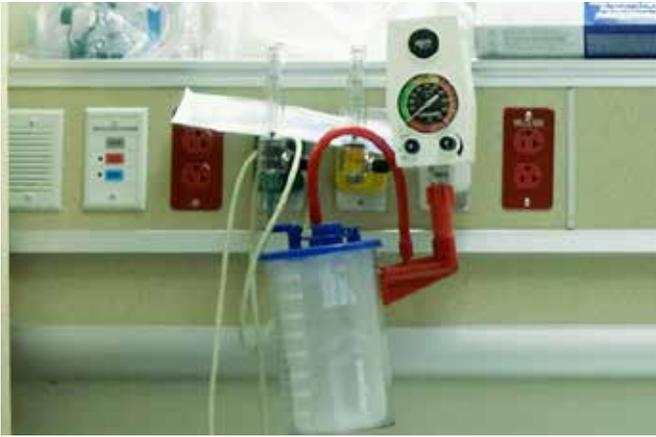
The new BeaconMedaes Series B Outlet Hook Plate features a retractable hook, allowing for the placement of wires and setup items without damage to the equipment or outlet for worry-free and dependable service.
